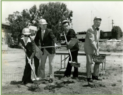
July 7, 1977 Groundbreaking - Arc Workshop
